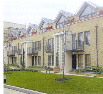
A well articulated roofline, a strong horizontal parapet and well proportioned fenestration all contribute to the quality of this scheme. Even the guttering and vents are used to punctuate the facade and contribute to the sense of proportion. Brightlingsea Place, Tower Hamlets. (p.74)
