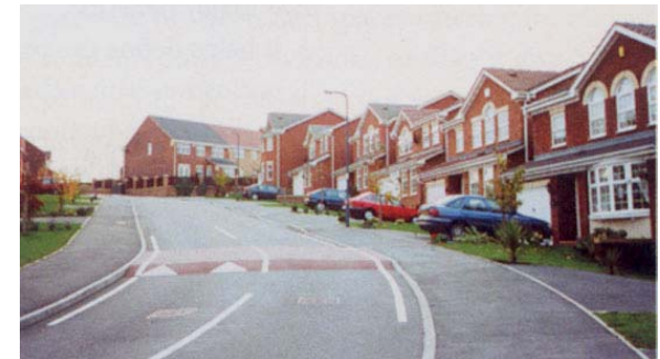
Front curtilage parking can result in over wide streets and the need for 'add-on' speed controls
