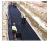
INSTALLING THE TANK MODULES
