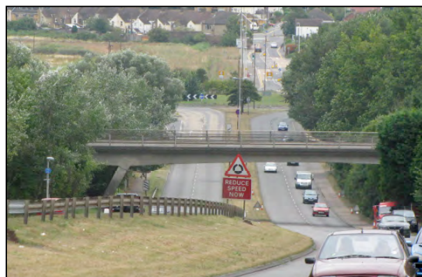
Figure 5.7: Upchat Road bridge
