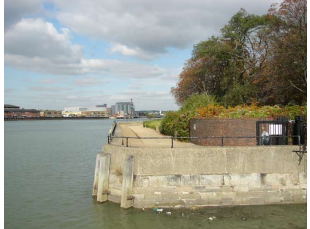
Gun Wharf Flood Defences
