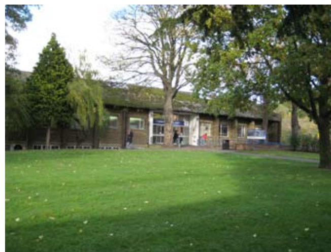
Some Low Quality Buildings
