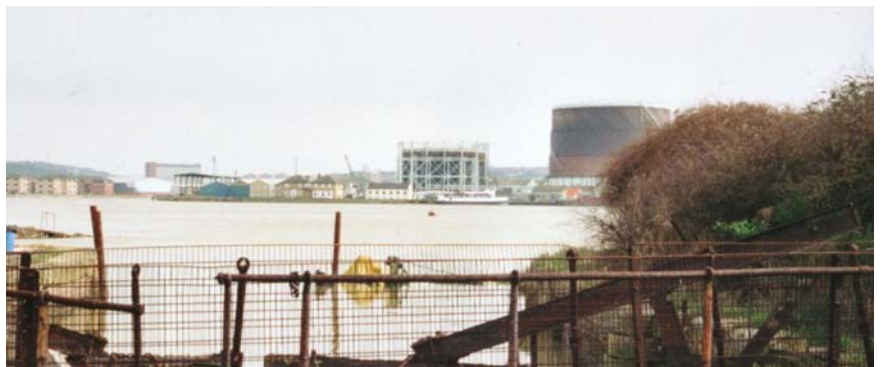
River Medway – View looking towards Rochester Riverside site from Strood
