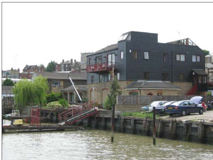
Conversion of former riverside warehouse for housing purposes with spectacular panoramic views of the river
