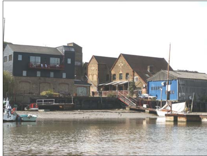
A 'jagged', interesting skyline created by the historic riverside buildings and warehouses
