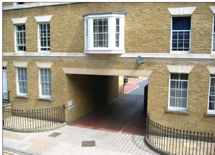
Carriage arch provides a solution to getting parking for houses off the High St and out of view
