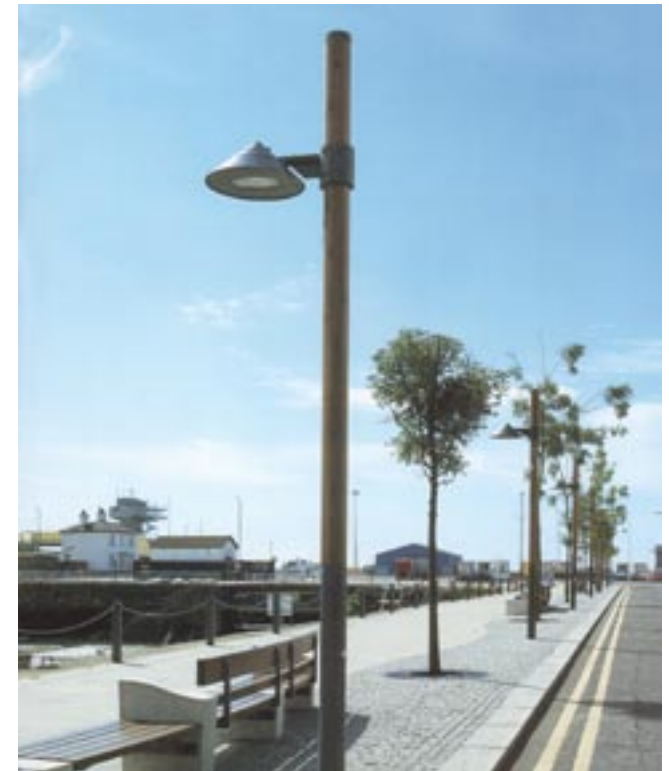
Lighting along a canal edge
