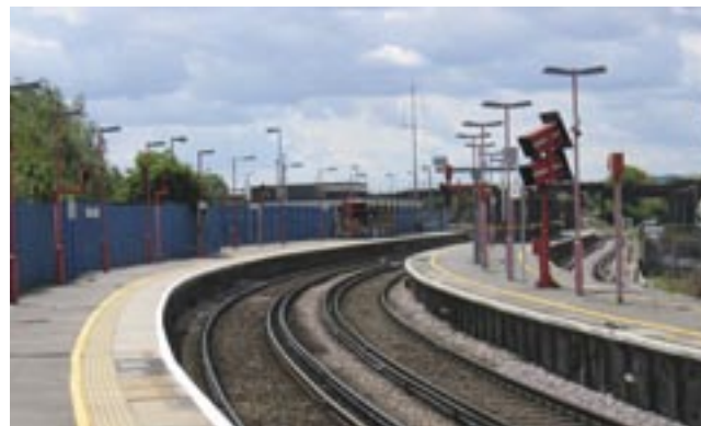
Railway line on the western boundary
