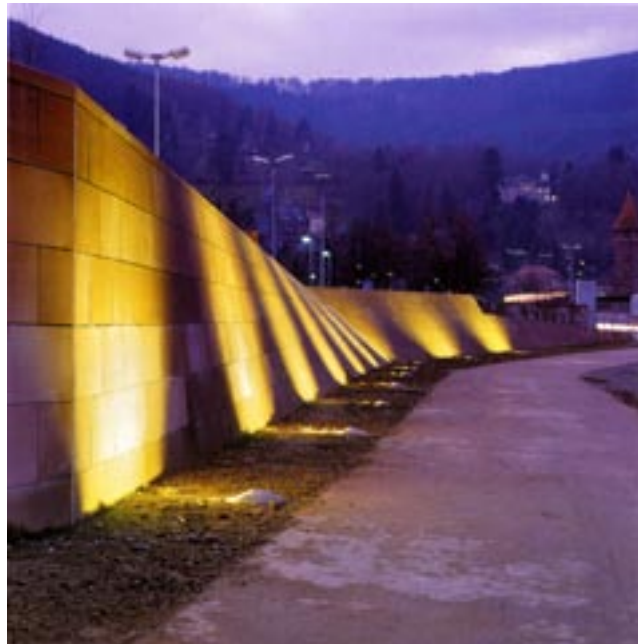
Lighting along a bank of flood protection
