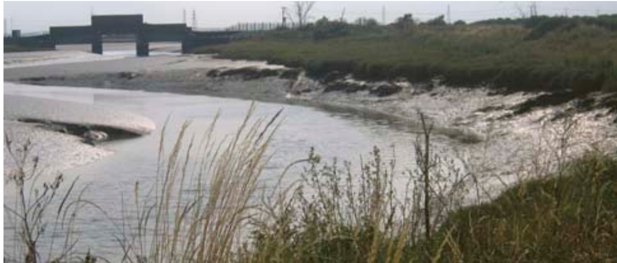
East Haven tidal control barrier
