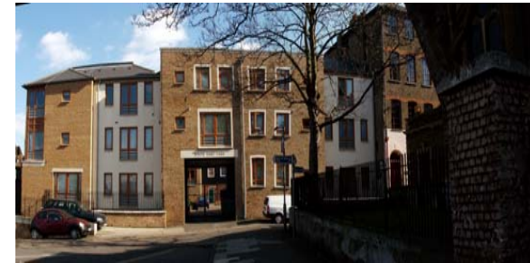
Example of modest backland development, Gravesend. This sort of scale and form is suitable for development sites within the City Wall Quarter.
