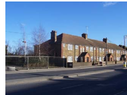
Low scale housing and vacant garage on Corporation Street.
