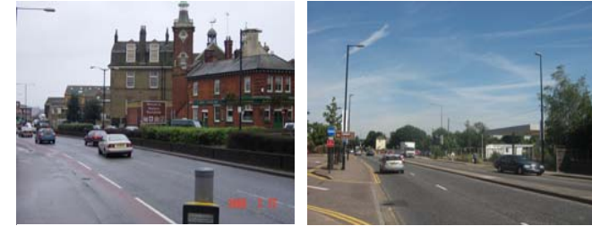
Corporation Street— an important gateway into Rochester. The dual carriageway severs connections between historic Rochester and planned development at Rochester Riverside.
