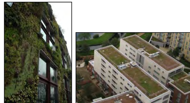
Figure 4.5: Green walls and roofs
