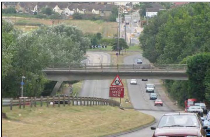
Figure 5.7: Upchat Road bridge
