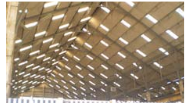
Roof structure inside the Covered Slip
