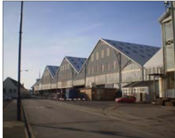
Covered Slip Buildings looking south
