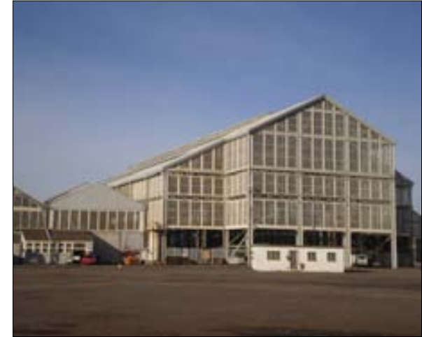
Photo showing the Covered Slip No. 7
