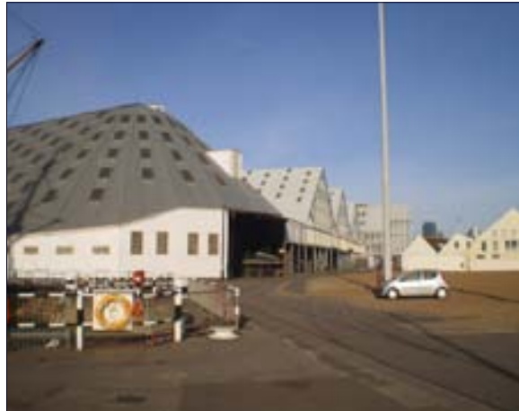
Covered Slip Buildings looking north
