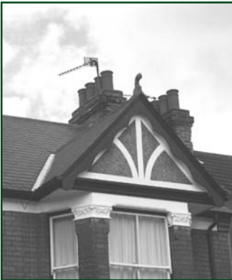
Good roof example
